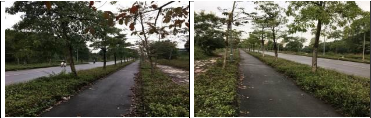
Rainwater drainage system is built submerged on the pavement
