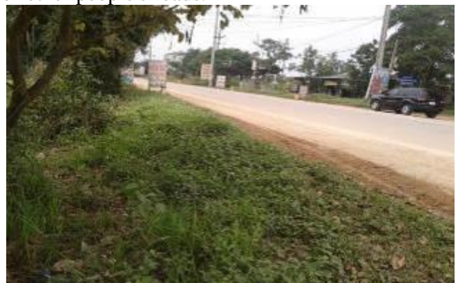
Figure 2.7: Existing Status of National Highway 21A
